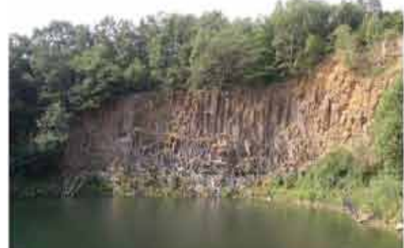
2: Quarry Pond with safety enhancements
